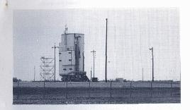
On RIGHT, you can now see the Polaris ground launching stands. The two light-gray service structures are used in the initial test launches. Once the reliability of the Polaris has been established here, further testing takes place at sea from the USS Observation Island. When reliability is obtained at sea from the surface vessel, Polaris missiles are placed in vertical missile launch tubes of one of the various nuclear submarines to undergo the underwater launch phase of the test program.
