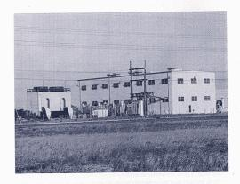
On LEFT you will see a two-story gray building with large outside plumbing. This is our liquid-oxygen-producing plant. Liquid oxygen, or LOX as it is commonly called, is the oxydizing agent used in combination with highly-refined kerosene to fuel such missiles as the Atlas and the Thor. The convenient on-Cape location saves transporting the very cold (-297.9 degrees Fahrenheit) LOX over public hierways.
